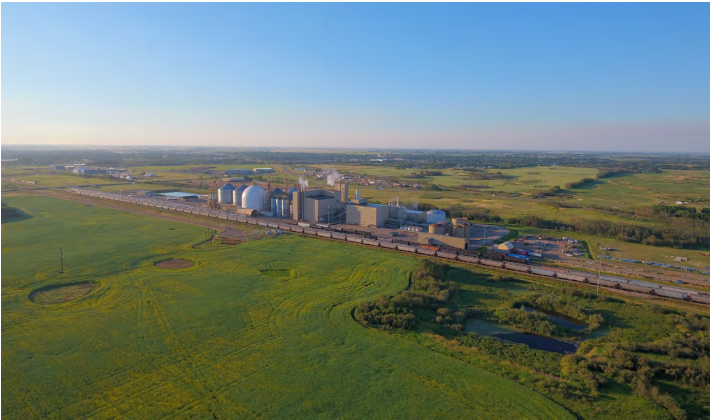
LDC canola crushing facility, Yorkton, Saskatchewan Photo credit: Louis Drefus Company
