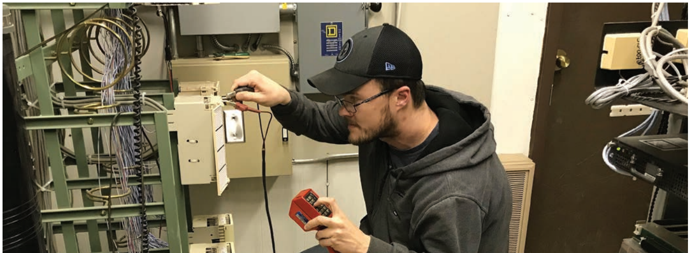
Keith Perras, Customer Service Technician, works on a maxTV Stream install.
