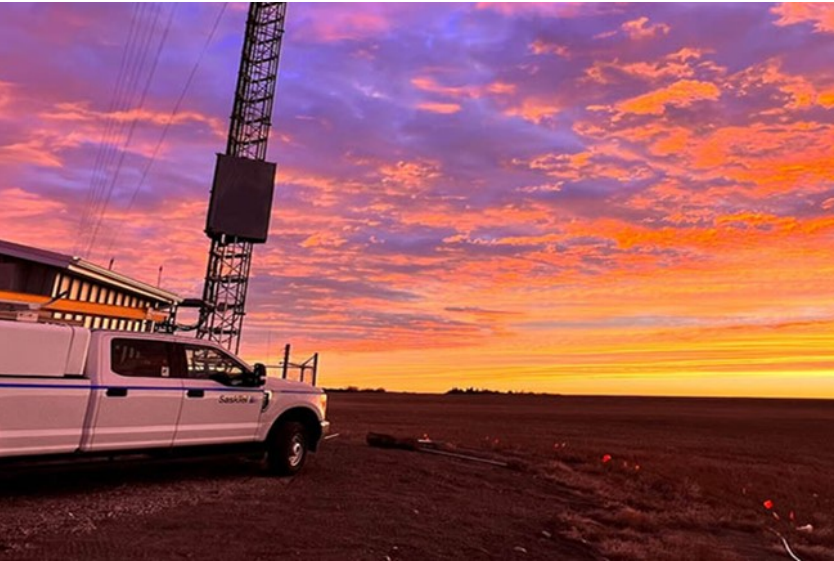
At the tower site, photo by Kevin Leek, SaskTel Trunking & Switching Technician
